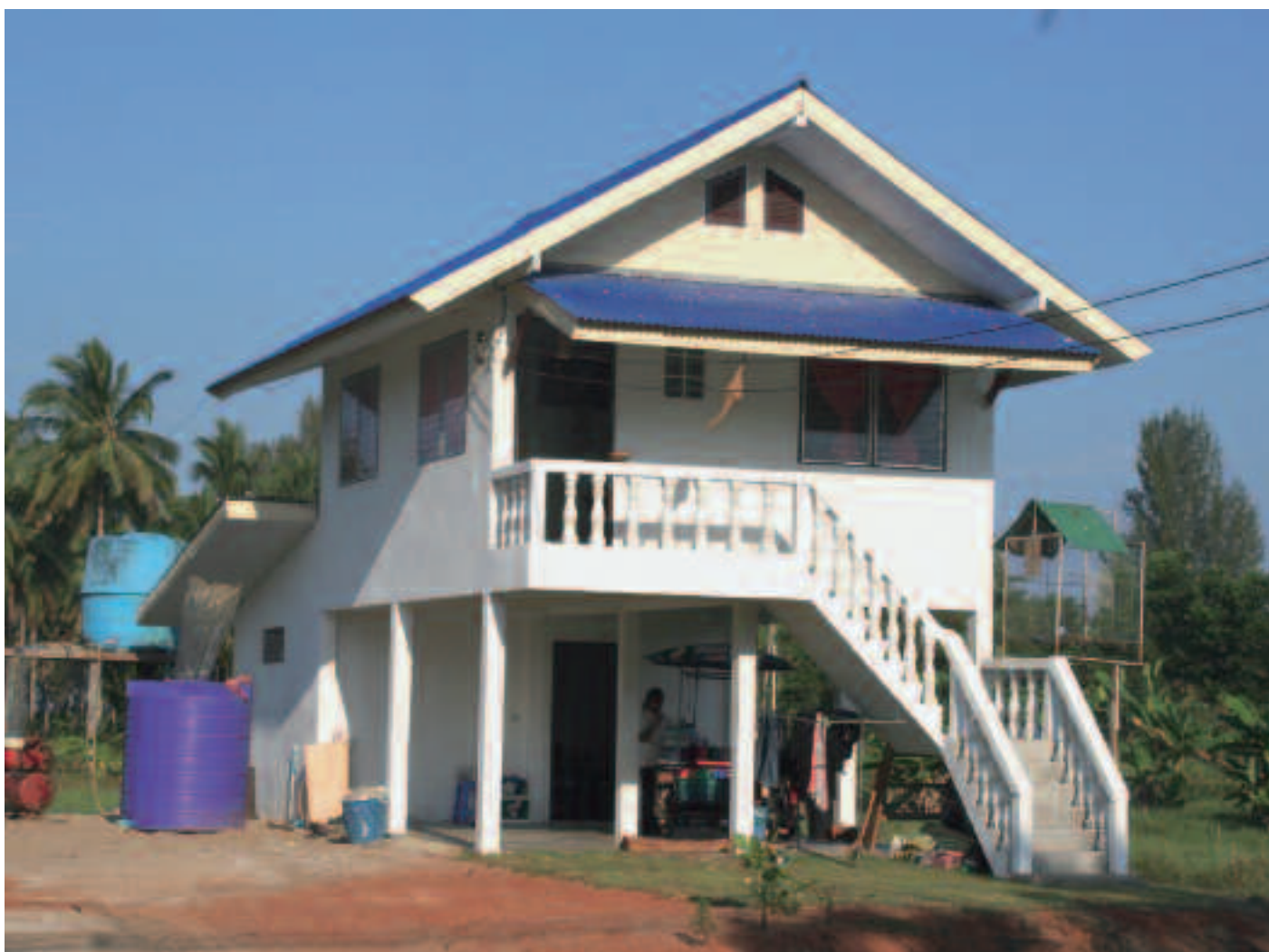
Building with an awareness of the risks: the newly-built houses in the tsunami area around Khao Lak, Thailand, are built on stilts. This allows the inhabitants to get to safety when the flood warning sounds. The measure is sustainable, provided the building regulations are complied with. Foto: T. Loster
